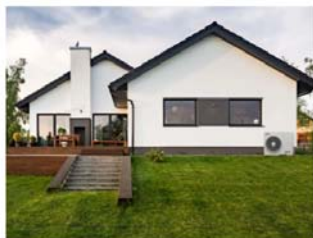
Air Source Heating
