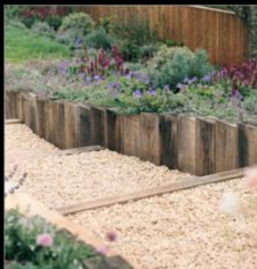
Hard Landscaping & Groundworks
