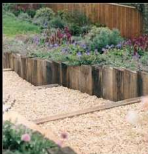
Hard Landscaping & Groundworks
