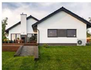
Air Source Heating
