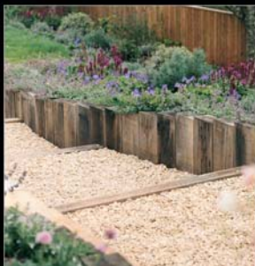
Hard Landscaping & Groundworks
