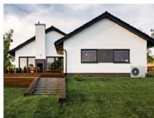
Air Source Heating
