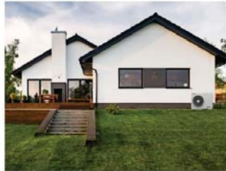
Air Source Heating
