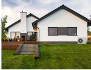
Air Source Heating
